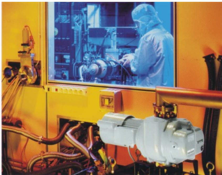
Pumping unit with roots pump for microelectronic application
